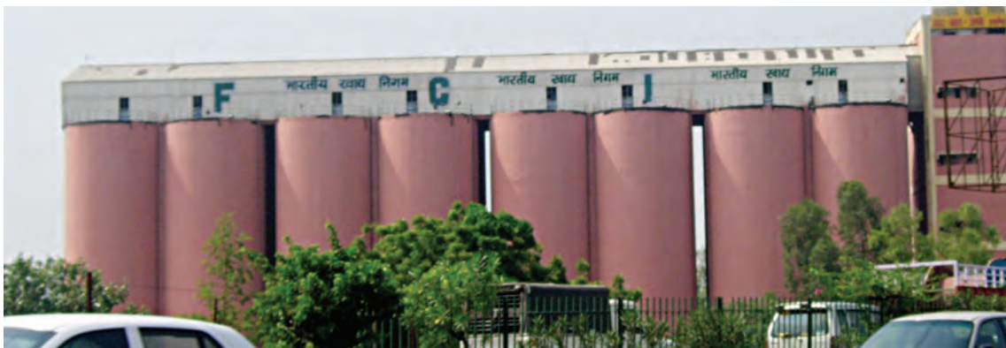
Fig. 1.10 (a) : Silos for storage of grains
