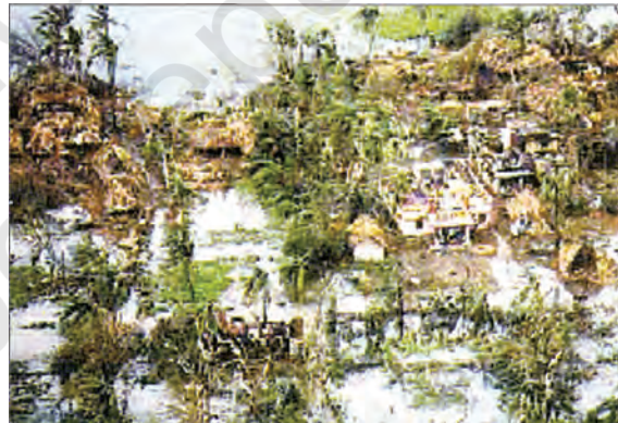
Destruction caused by a cyclone
