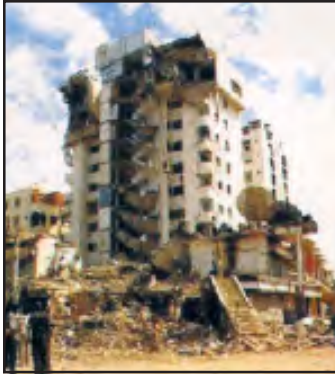
Fig. 3.3a: Destruction caused by an Earthquake in Gujarat
